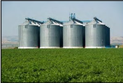
Grain Storage Facility
